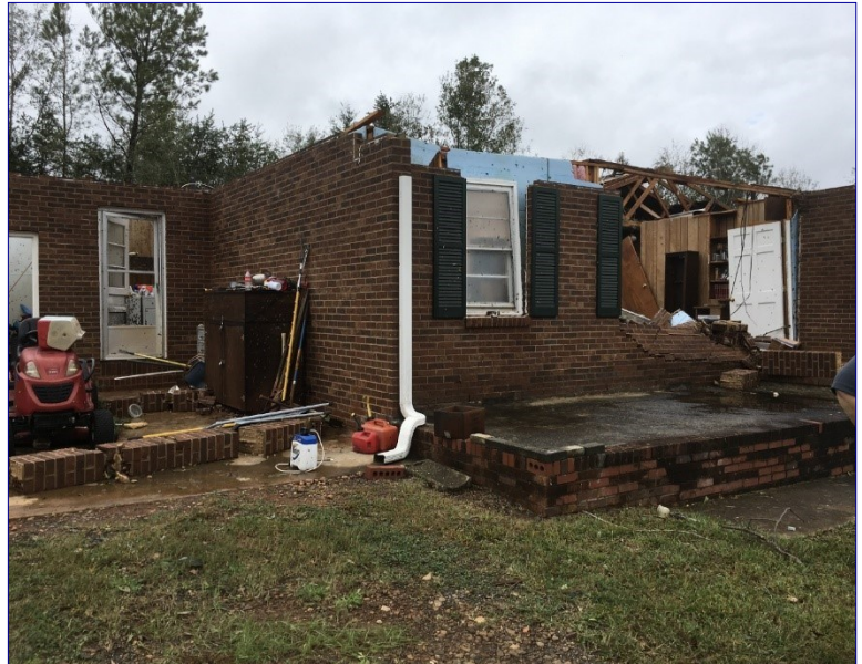
Fig 5. An EF2 tornado blew roofs from homes near Norris, SC on 8 October 2017
