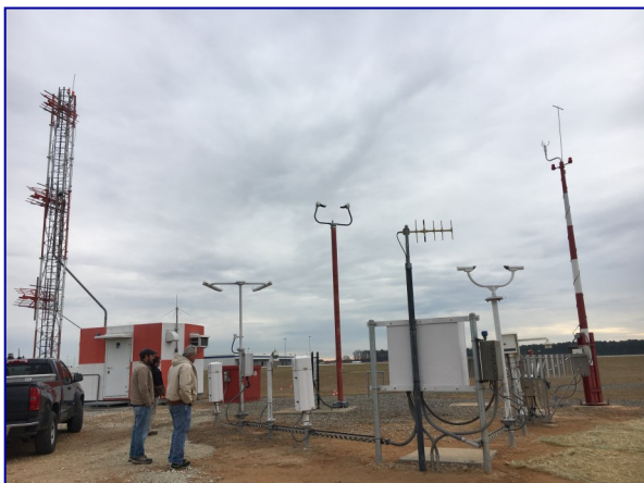
NWS technicians inspect the ASOS at the GSP Int'l Airport.
