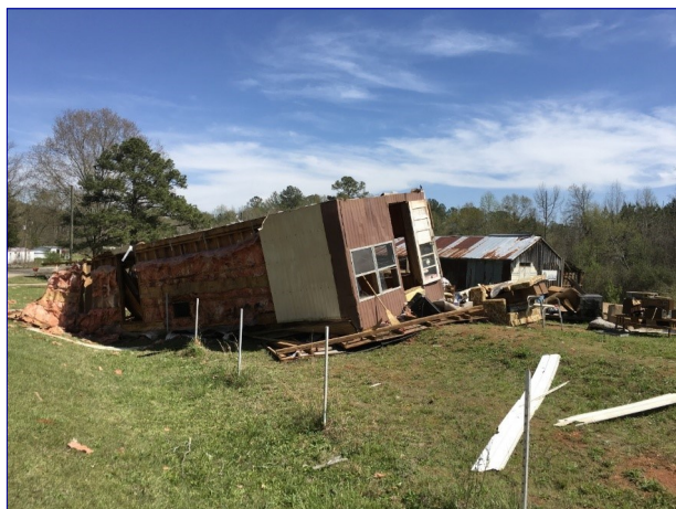
Fig 3. Weak tornadoes flipped mobile homes in Union County, SC on 3 April 2017.
