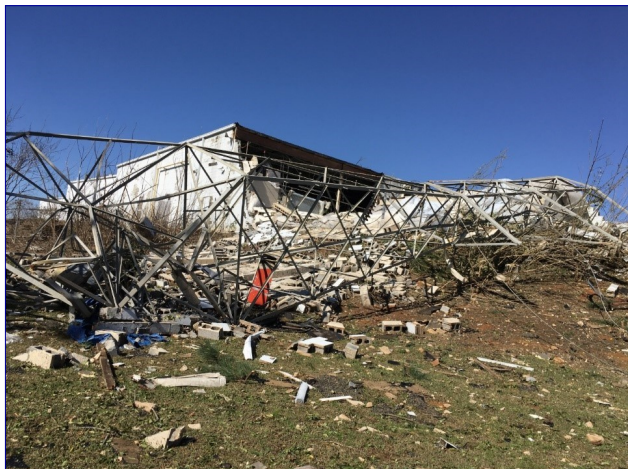
Fig 8. A high voltage tower was toppled by an EF2 tornado along Business 85 on the north side of Spartanburg, SC on 17 October 2017. Part of the warehouse building in the background was also destroyed.
